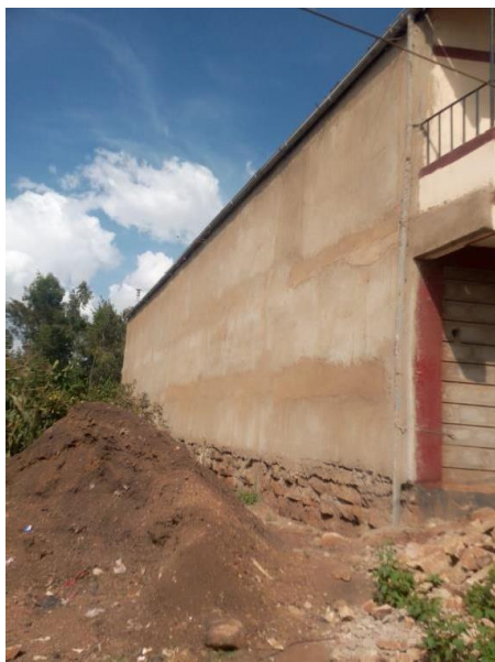
The right side part of the building after plastering
