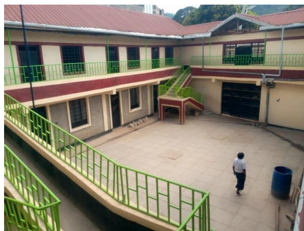
The compound after installation of paving slabs
