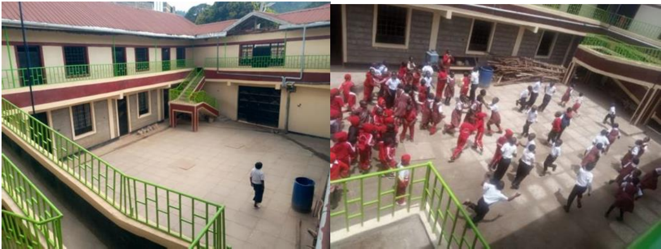
The compound after installation of paving slabs Children happily playing in the very impressive compound
